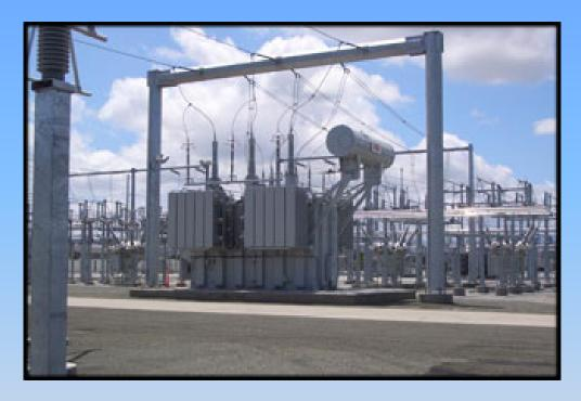
A distribution substation is a system of transformers, meters, and control and protective devices. At a substation, transmission line voltage is reduced to lower voltages for distribution to residential, commercial, and small and medium industrial customers.
