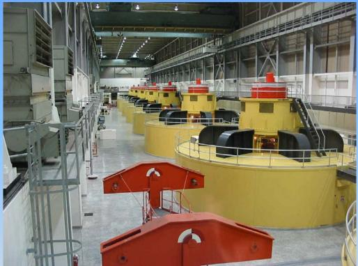
Falling water strikes a series of blades attached around a shaft which converts the kinetic energy to mechanical energy, and causes a turbine to rotate. The shaft is attached to a generator, so that when the turbine turns, the generator is driven. The generator converts the turbine's mechanical energy into electric energy.
