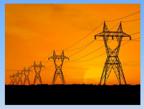
Grid transmission lines, usually supported by tall metal towers, carry high voltage electricity over long distances. The BC Hydro high-voltage transmission system consists of 18,286 kilometres of transmission lines, operating at voltages from 60 kV to 500 kV.
